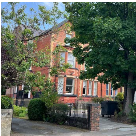
Residential properties along Park Road
